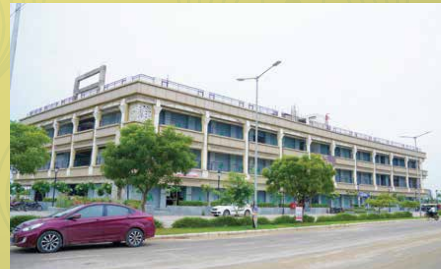
GYC GALLERIA SHOPPING COMPLEX
