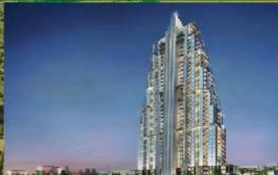
RAHEJA OMA (Under Construction)
