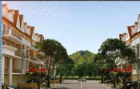
RAHEJA AYANA (Under Construction)
