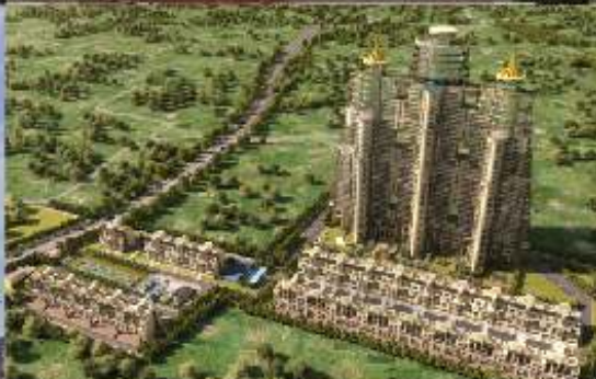
RAHEJA REVANTA (Under Construction)
