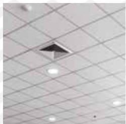
CEILING GRID FALSE CEILING
