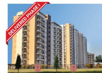
SECTOR 37C, GURGAON DWARKA EXPRESSWAY
